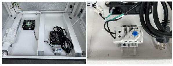
Verify that the temperature-control switch it set to 30°C (as shown in the image on the right).
