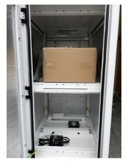
Line up battery with the mounting holes on the cabinet
