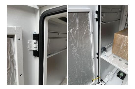
Remove the door and replace with the AC/door unit. Reattach the hinge and ground cable. Connect the AC power cable to the AC unit and plug in the power cable to the power strip.
